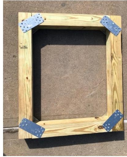
Figure 7: 16-gage galvanized steel tie-plates Figure 8: Assembled wooden platform frame
