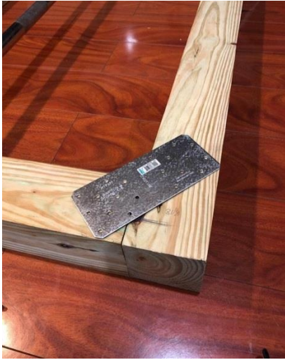
Figure 7: 16-gage galvanized steel tie-plates Figure 8: Assembled wooden platform frame
